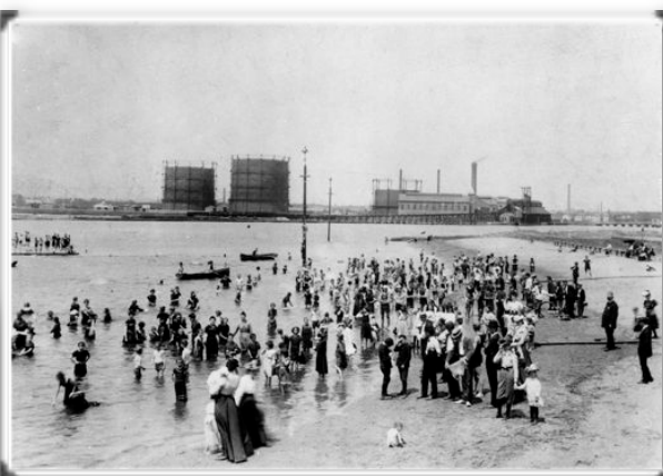
Bathers at Magazine Beach, 1906. Note the wharf, plant, and gas holders of the Brookline Gas Co., with the River Street Bridge on the extreme right. Coal was brought in by barge and heated in sealed retorts to drive off the gas. The gas was stored in the iron tanks. Description courtesy of Charles Sullivan. Photo, gift of Walter L. Colburn. Courtesy of Cambridge Historical Commission.
